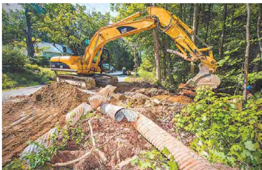
Culvert upgrade work in-progress on Dunbarton Center Road prior to its being resurfaced. Photo courtesy of Eric Anderson.
