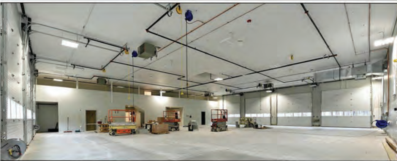
Fire Equipment Bays Public Safety Center
