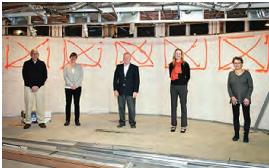
Library Trustees & Library Director in front of the window area to be created in the Bow Rotary Community Room in the Lower Level of the Library. The orange "x's" indicate where the concrete foundation needs to be cut for the new windows. Expected completion date for the Lower Level space is early February 2017. From left to right: David Withers; Christine Carey, Tom Ives, Lori Fisher (Director), and Benette Pizzimenti. Absent: Trustee Peirce Hunter. Photo by Eric Anderson.
