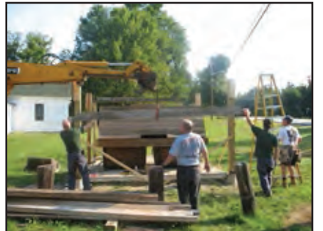
The Southwest Beam is Placed and Secured
