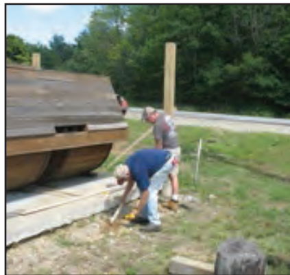
Plumbing the Vertical Pressure Treated Beams
