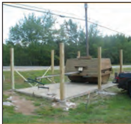
Plumbing the Vertical Pressure Treated Beams
