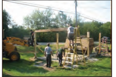
The Northeast Beam is Placed and Secured
