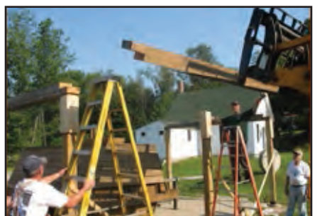
The Southwest Interlocking Side Beams are Placed
