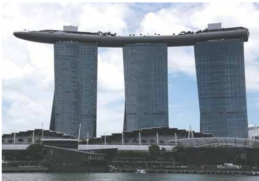
The Marina Bay Sands Hotel and Casino in Singapore cost $8 billion to build and features the unique SkyPark atop the three towers.
